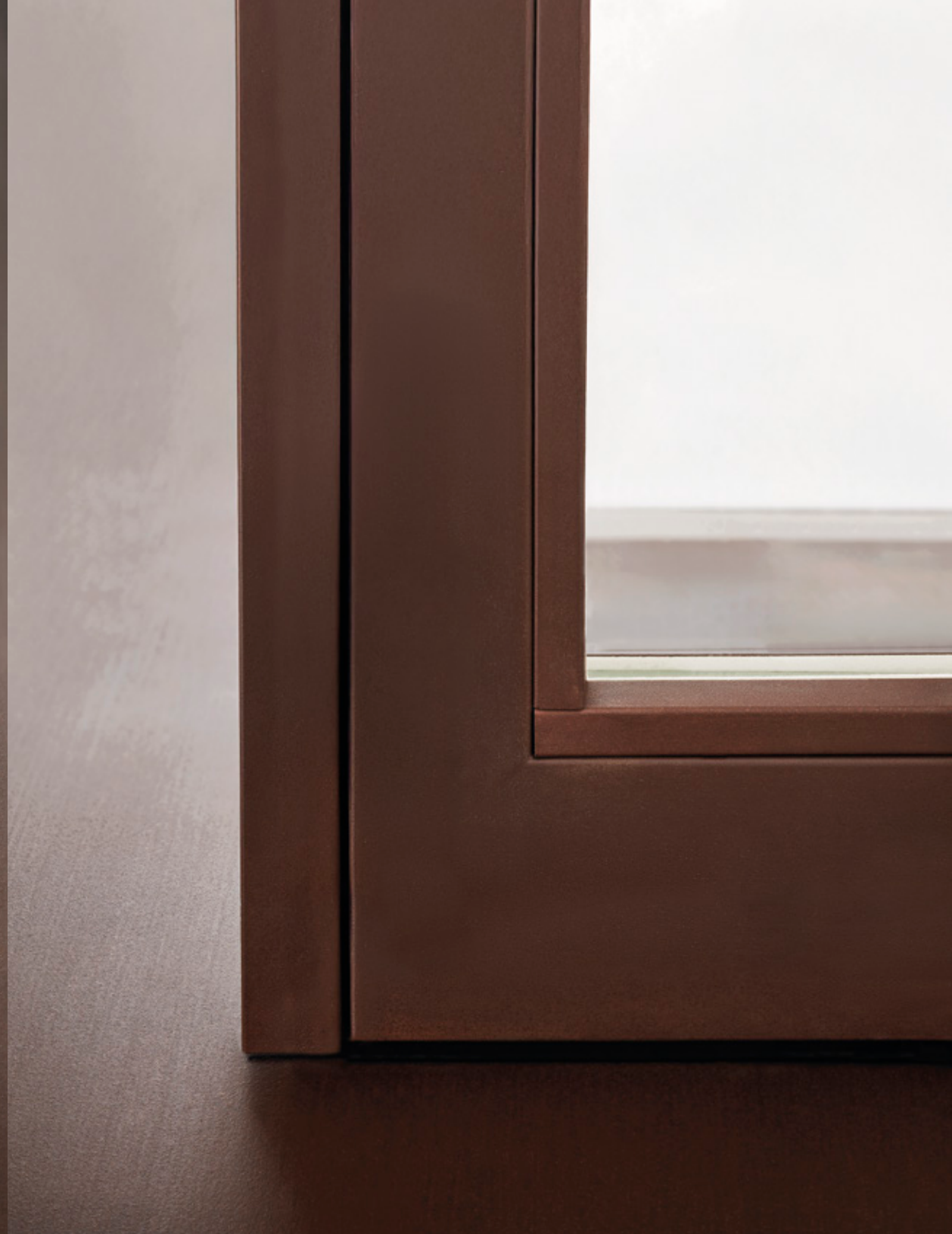
SA-AF - corten steel internal view
